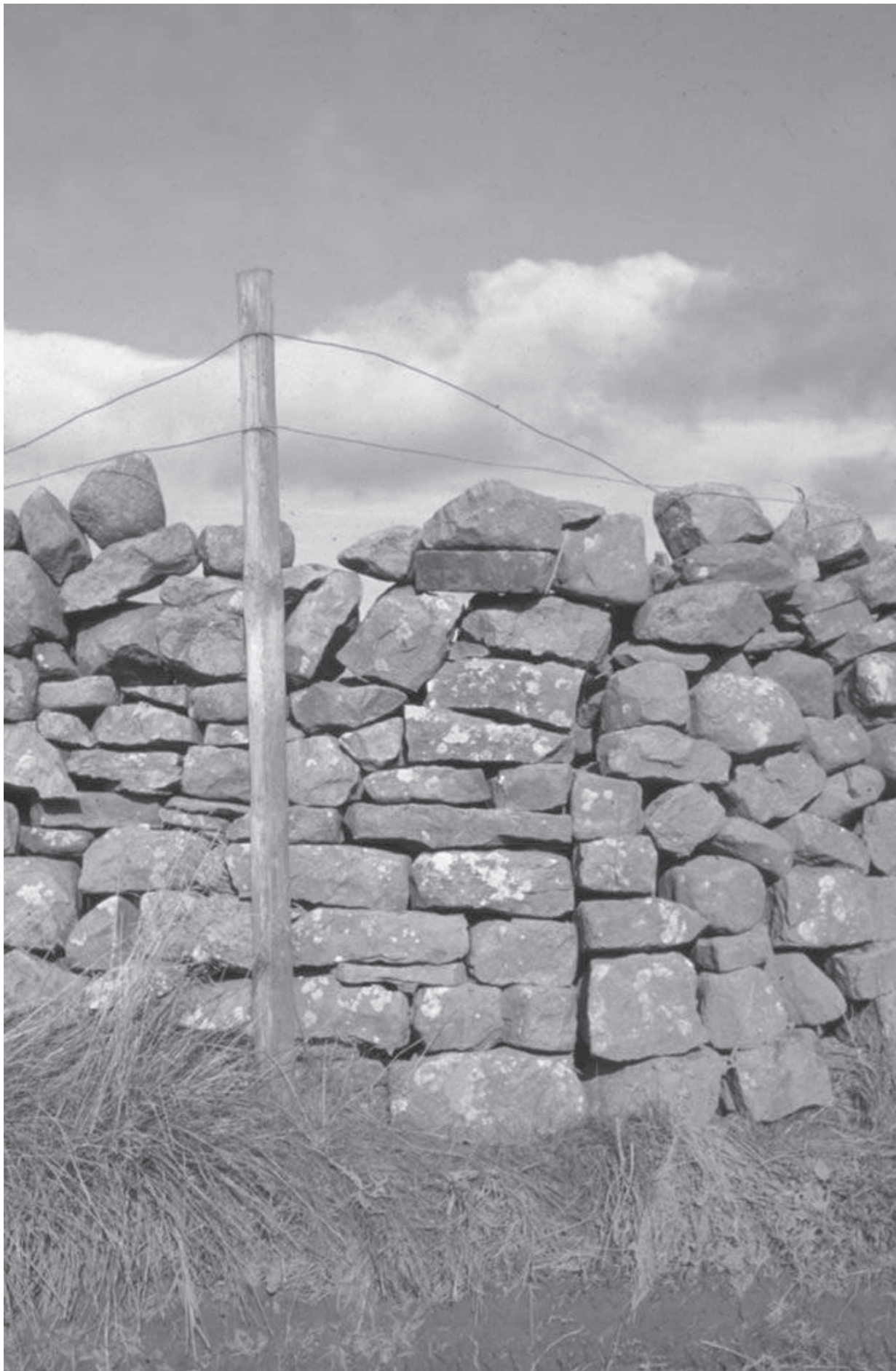
Figure P3 A “butt-joint” in a field wall, near Grinton, Swaledale
