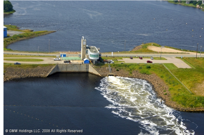
Zajezitvena plimska HE Annapolis Royal Generating Station (Can)
