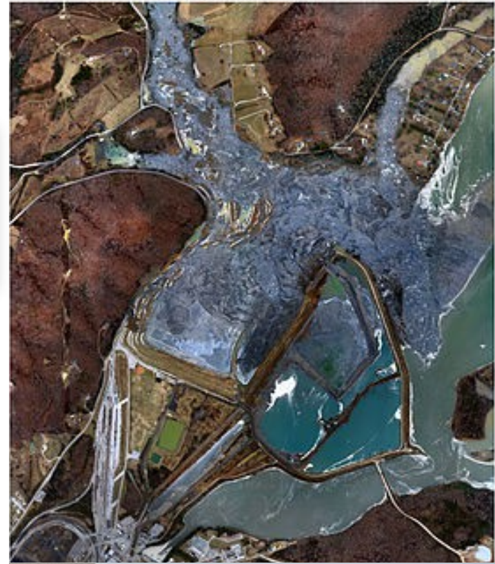
Aerial Image Of Kingston Ash Slide 12/23/08
